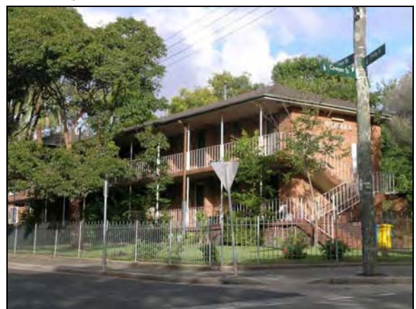
Photograph 4: Two (2) storey building, as viewed from the corner of Elger and Cowper Streets.
