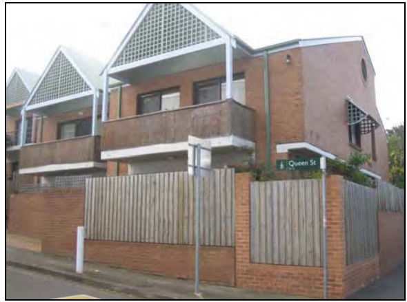
Photograph 16: Development to the south, as viewed from the corner of Queen and Bay Streets.
