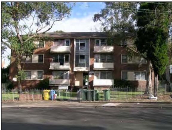
Photograph 1: Indicative three (3) storey building, as viewed from Elger Street.
