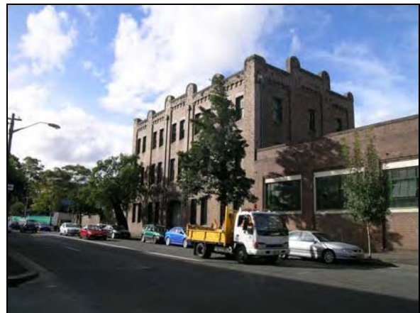
Photograph 12: City of Sydney Depot building to the east of the site.
