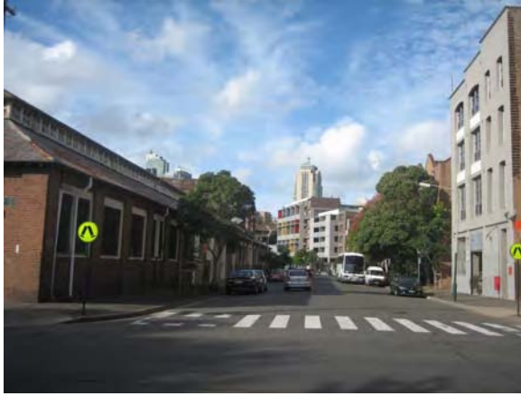
Photograph 13: Streetscape view of Macarthur Street as viewed from the corner of Bay Street facing east.
