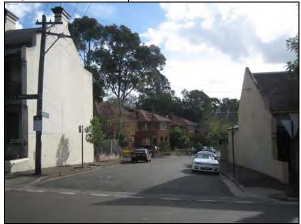
Photograph 22: Example of development to the west of the site on Phillip Street, as viewed from the corner of Cowper Street.
